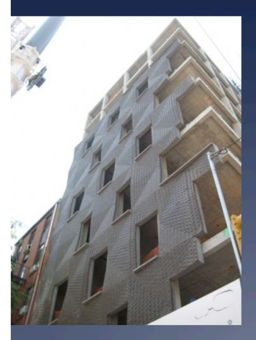
Bonded to a precast concrete backing
