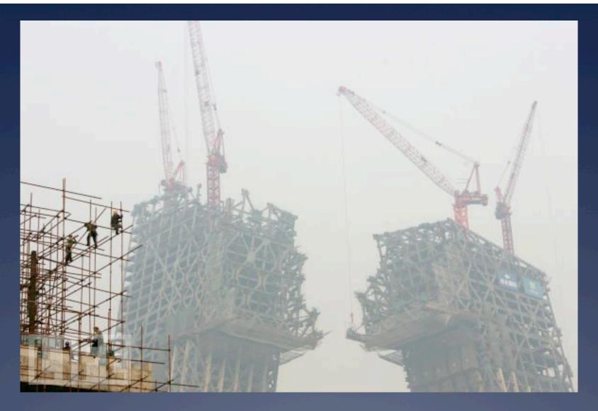
"Soft" connection at first, made at night when steel was uniformly cool, stress monitors
