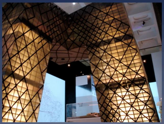
Instead of increasing the weight of each steel diagonal...add more where needed, take away where not... pattern informed by principle
