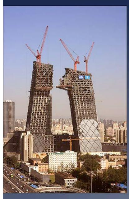
Counterbalanced with a mat foundation weigh 364,000 tons
