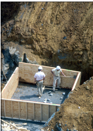
Positioning prefab column pad forms
