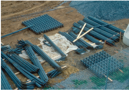
Rebar kit for column pads
