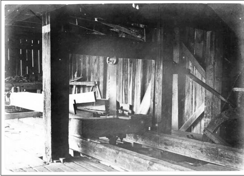
Fig. 8. Kanode Sawmill, 1901, showing water-driven frame or "Muely" saw outside Blacksburg, VA (VT ImageBase [ http://imagebase.lib.vt.edu/ ]) housed and operated by Digital Library and Archives, University Libraries; scanning by Digital Imaging, Learning Technologies, Virginia Tech [ http://spec.lib.vt.edu/imagebase/localhistory/full/BI-6.jpeg ]). Used with permission.
