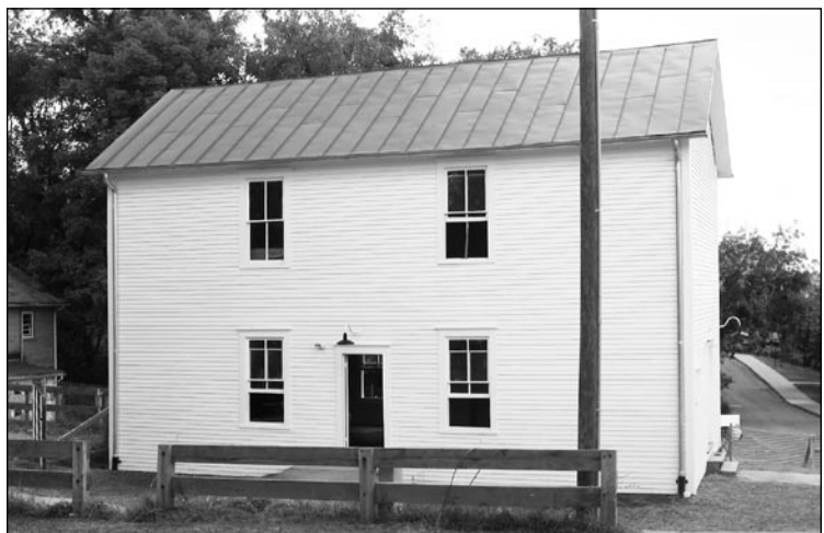
Fig. 9. Front of Odd Fellows Hall, restored 2007 (Photograph courtesy of the Blacksburg Museum).
