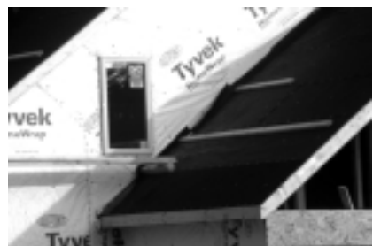
Housewrap, taped window joint over OSB. Allegheny St. Houses 1999
