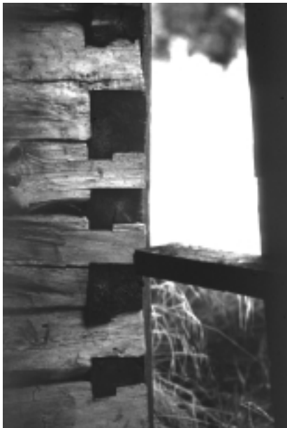
Lock joint in squared log construction, Embarrass, Minn. 1913
